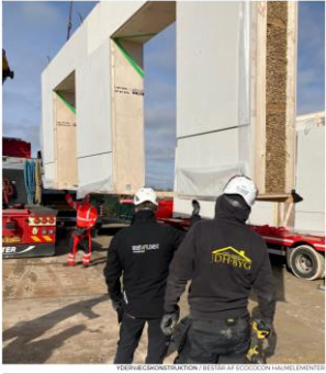
YDERVEKONSTRUKTION: BESTÅR AF ECOCOCON HALMELEMENTER Fire resistance classification: (Valid for the section on internal wall face covered with clay base plaster) REI 120 / REI 120 / REW 120
